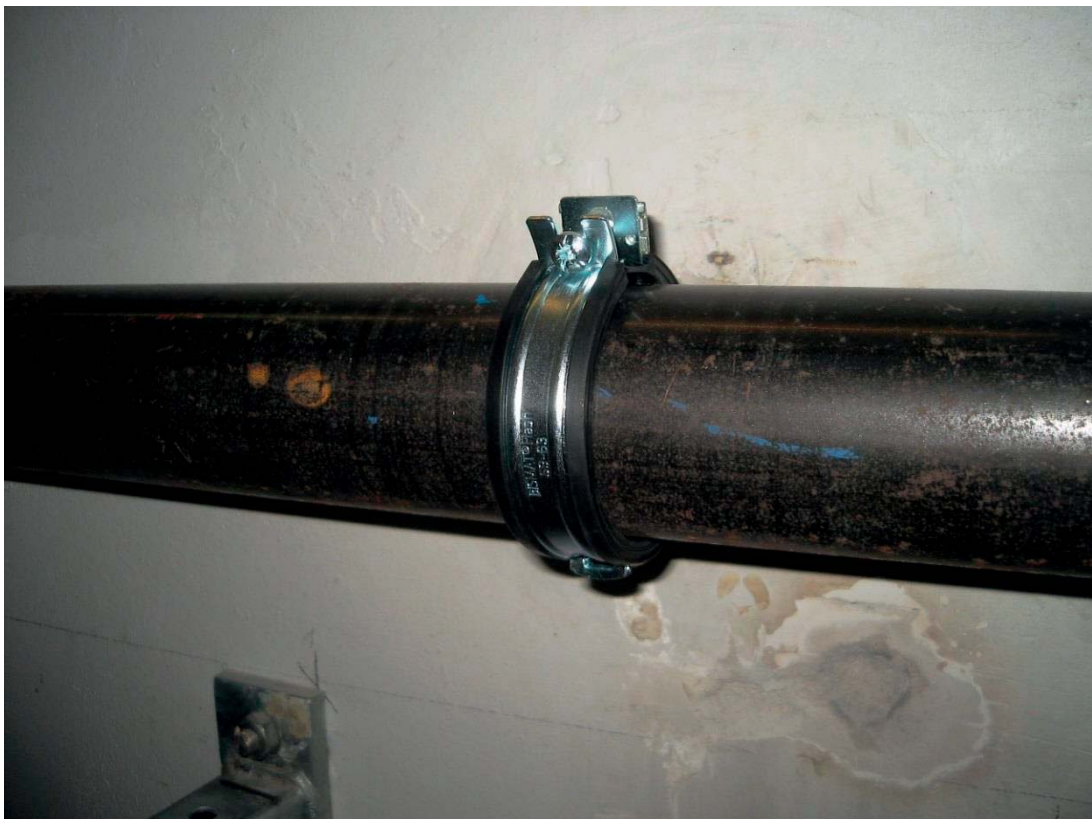
Fig. 2: Meas. 3: BISMAT® Flash, 2" (59 - 63mm), connection M8/10, with EPDM-rubber (20 x 4,20 mm)
