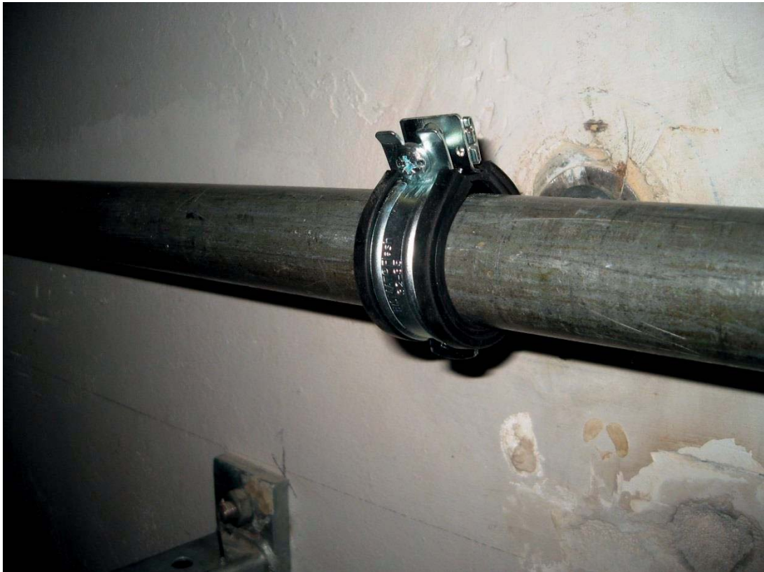
Fig. 1: Meas. 2: BISMAT® Flash, 1" (32 - 35mm), connection M8/10, with EPDM-rubber (20 x 4,20 mm)
