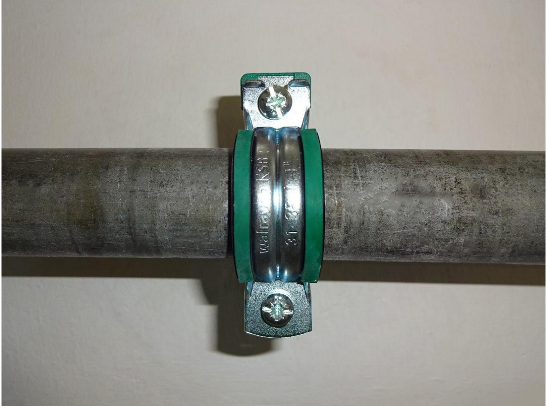
Fig. 1: Meas. 2: KSB2 two-screw-clamp, 1" (31 - 35 mm), connection M8/10, with EPDM-rubber (20 x 3,70 mm)
