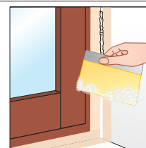
Finish the sealing with a wet spatula
