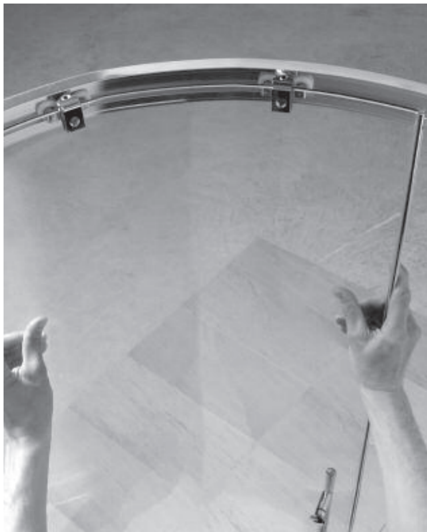
10 Working from inside the enclosure set the doors into the top rail. Double rollers on top
