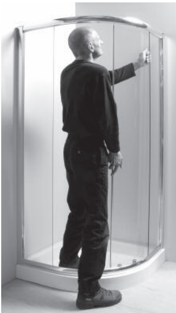
9 Fit moving panels B into frame.
