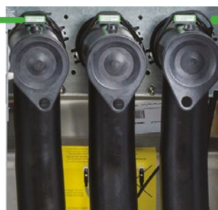
TH110 mounted on cable termination
