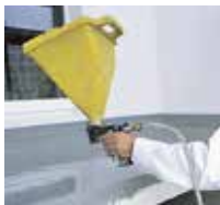
10 ... soffiare Triflex Micro Chips.
