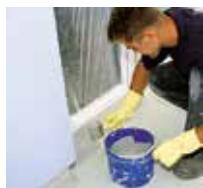
12 Applicare la sigillatura Triflex Cryl Finish 205 e ...
