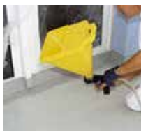
13 ... soffiare Triflex Micro Chips.
