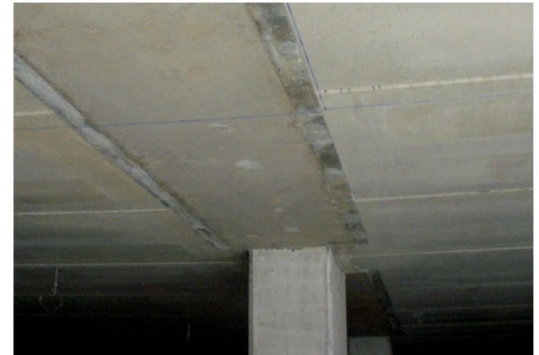
Trave NPS® Rei S con forometrie – NPS® Rei S Beam with bore holes
