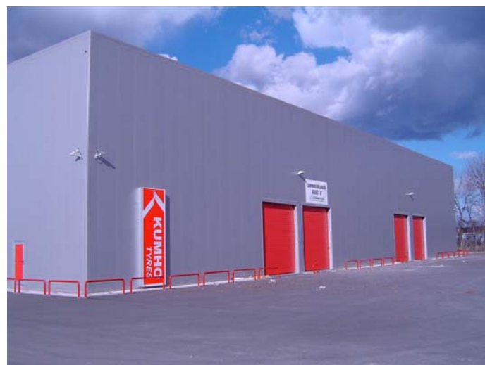
Pannelli montati in Slovenia
