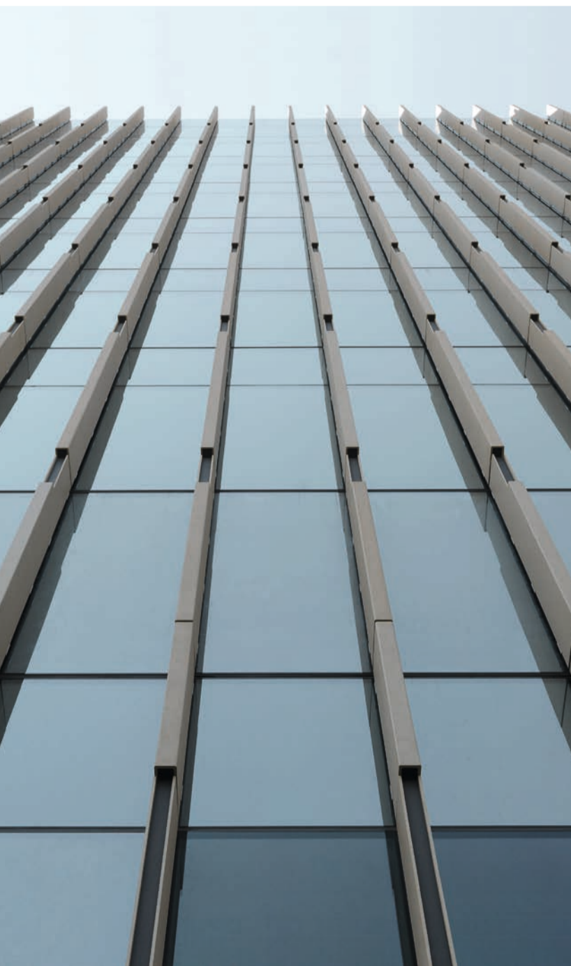
Boston University CENTER FOR INTEGRATED LIFE SCIENCES AND ENGINEERING formparts, concrete skin / sandstone, liquid black / ferro, ferro light PAYETTE
