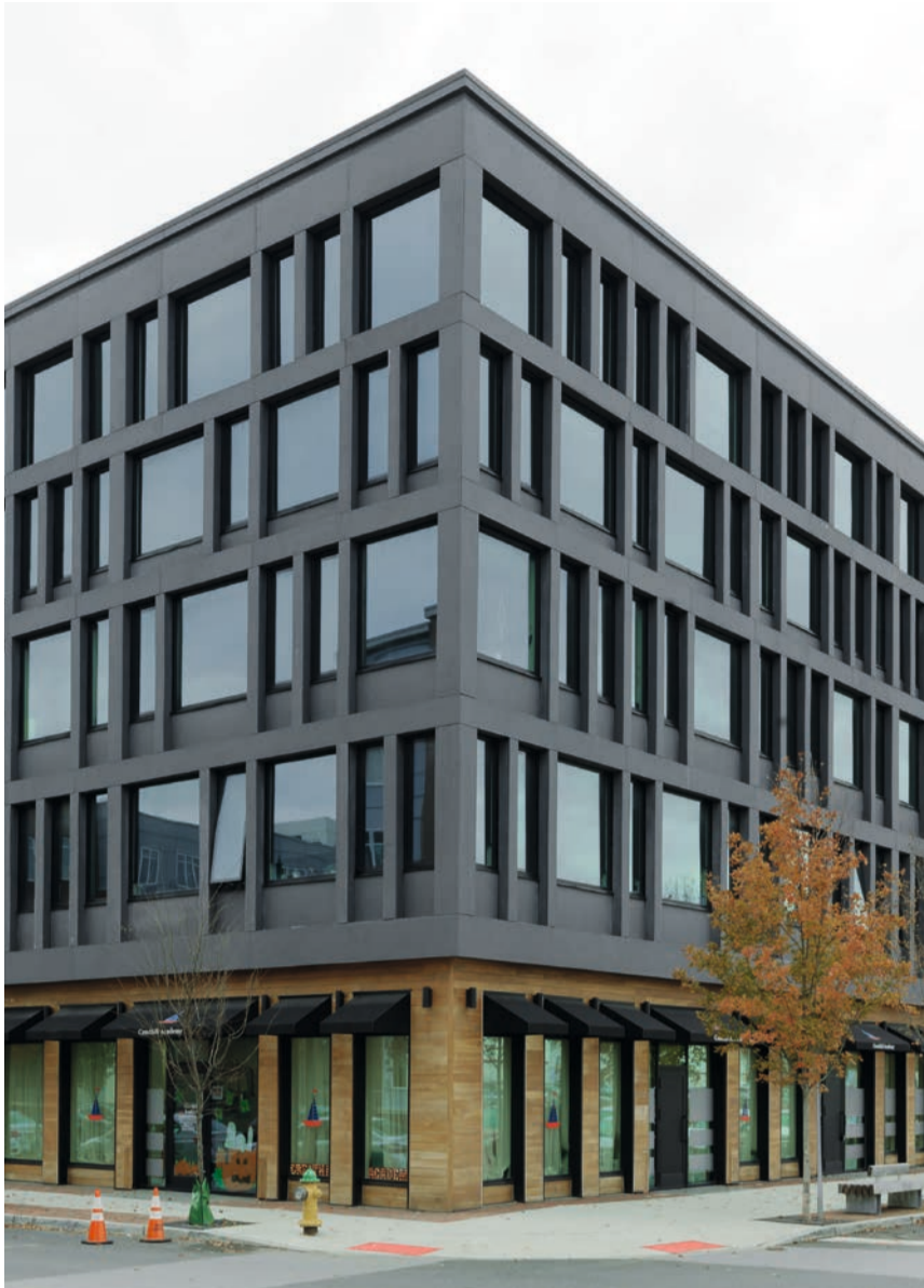
Harrison Common New Jersey concrete skin / off-white, liquid black / ferro light MINNO & WASKO ARCHITECTS & PLANNERS
