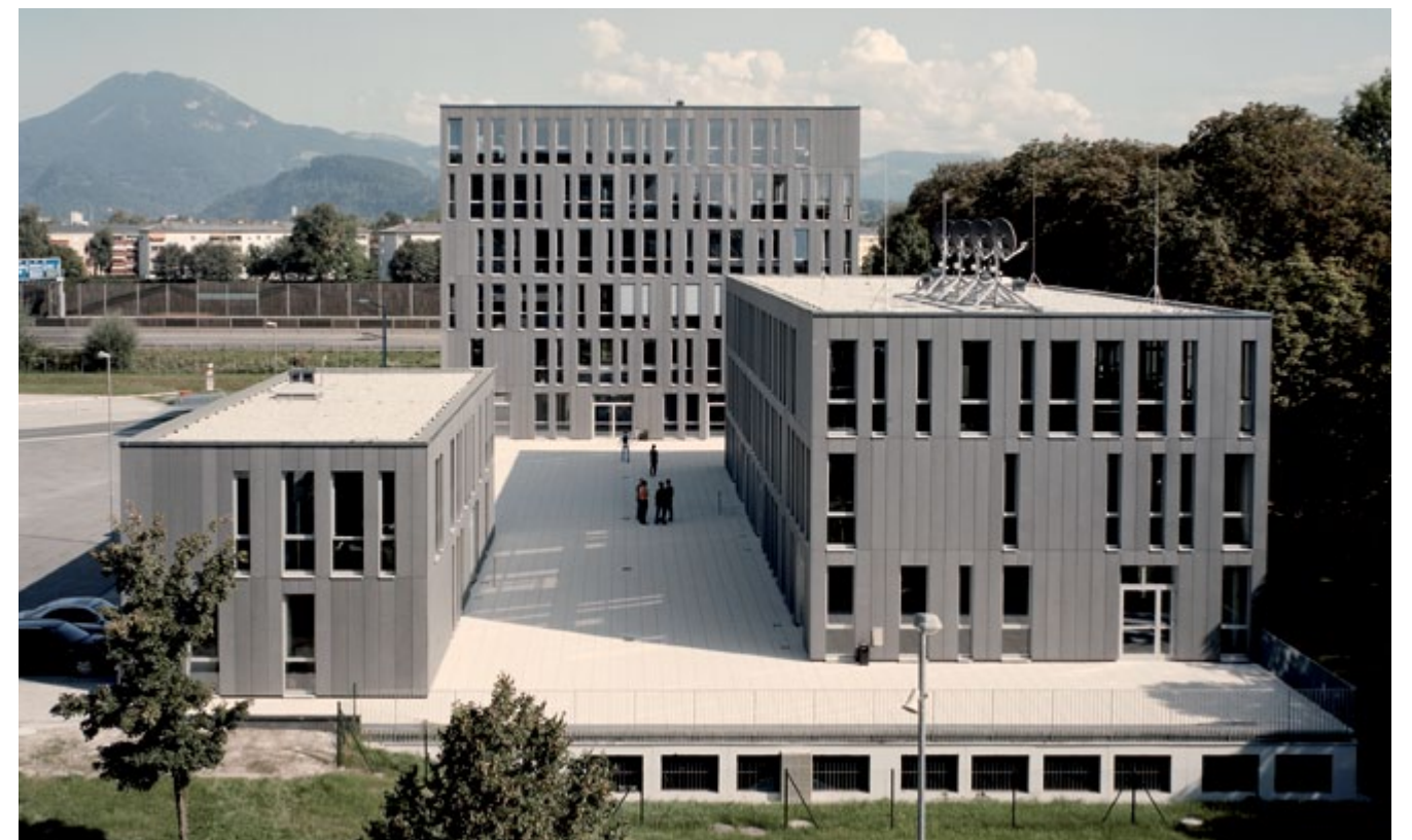
Office Building Salzburg, AT | Schuster Architects Salzburg, AT | 1,100 m 2 fibreC facade | anthracite | FE | adhesive Bürogebäude Salzburg, AT | Schuster Architekten Salzburg, AT | 1,100 m 2 fibreCFassade | anthrazit | FE | geklebt
