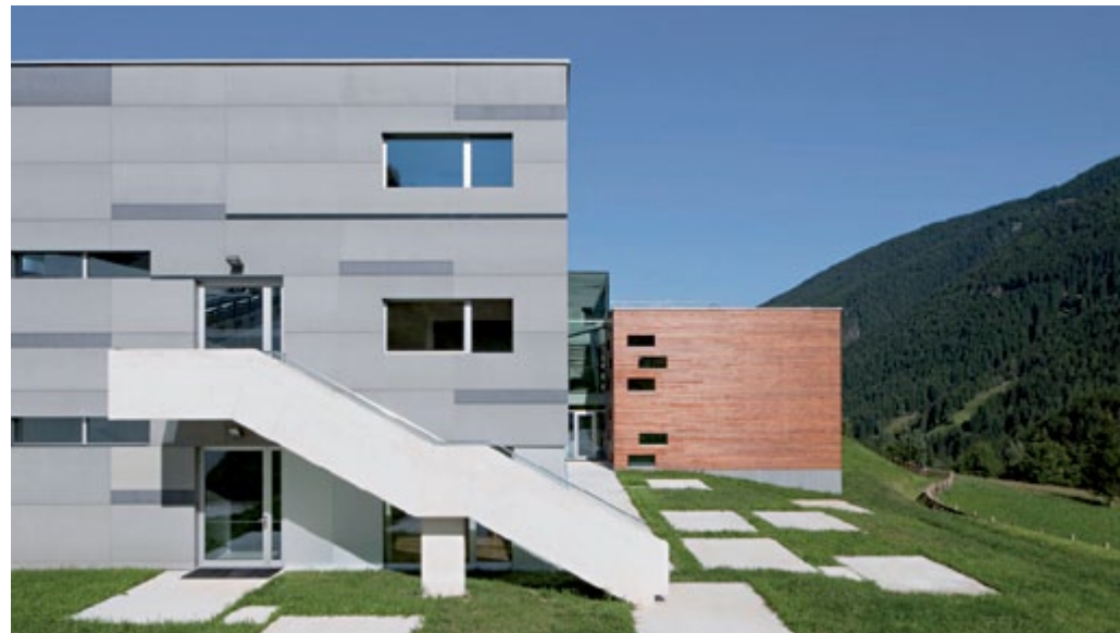
Primary School St. Walburg, IT | S.O.F.A. Architects Vienna, AT | 1,200 m 2 fibreC facade | silbergrey & anthracite | FE | riveted Grundschule St. Walburg, IT | S.O.F.A. Architekten Wien, AT | 1,200 m 2 fibreC Fassade | silbergrau & anthrazit | FE | genietet
