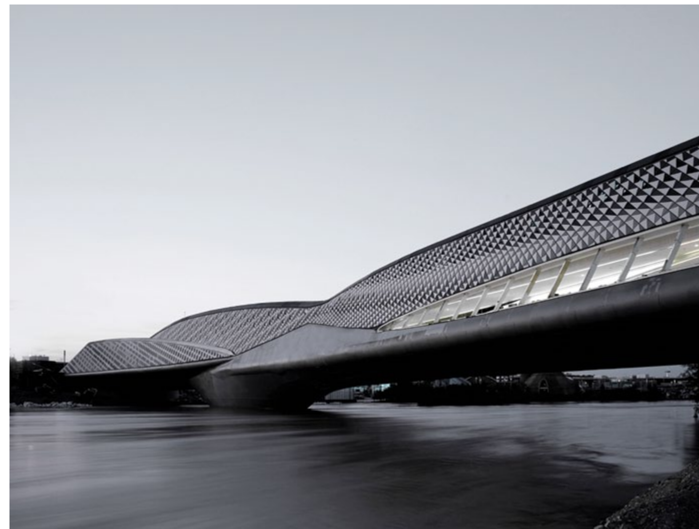
Zaragoza Bridge Pavilion for EXPO 2008 Zaragoza, ES | Zaha Hadid Architects London, UK | 11,500 m 2 fibreC facade | grey shades | FE | riveted Zaragoza Bridge Pavilion für die EXPO 2008 Saragossa, ES | Zaha Hadid Architekten London, UK | 11.500 m 2 fibreC Fassade | Grautöne | FE | genietet
