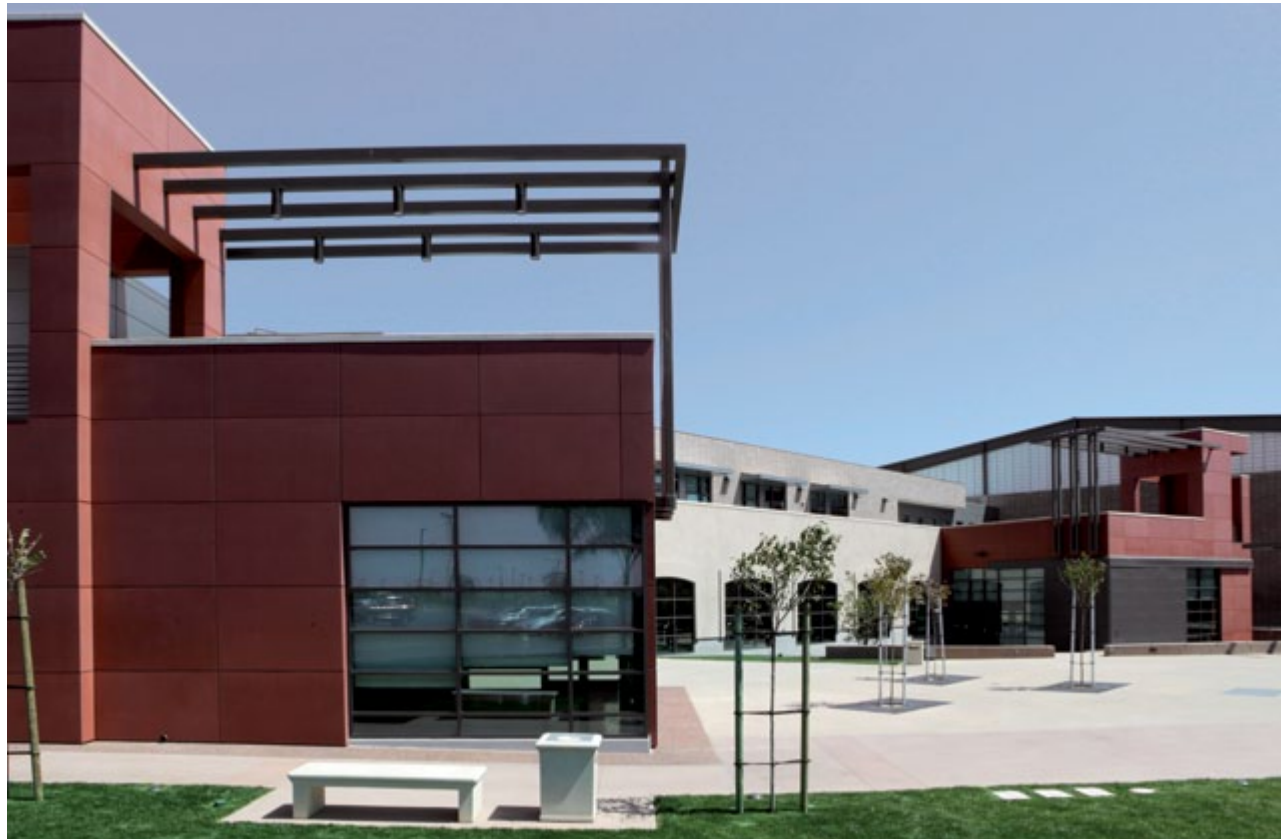
Miramar College San Diego, US | Carrier Johnson Architecture San Diego, US | 900 m 2 fibreC facade | terracotta | MA | screwed Miramar College San Diego, US | Carrier Johnson Architektur San Diego, US | 900 m 2 fibreC Fassade | terracotta | MA | geschraubt
