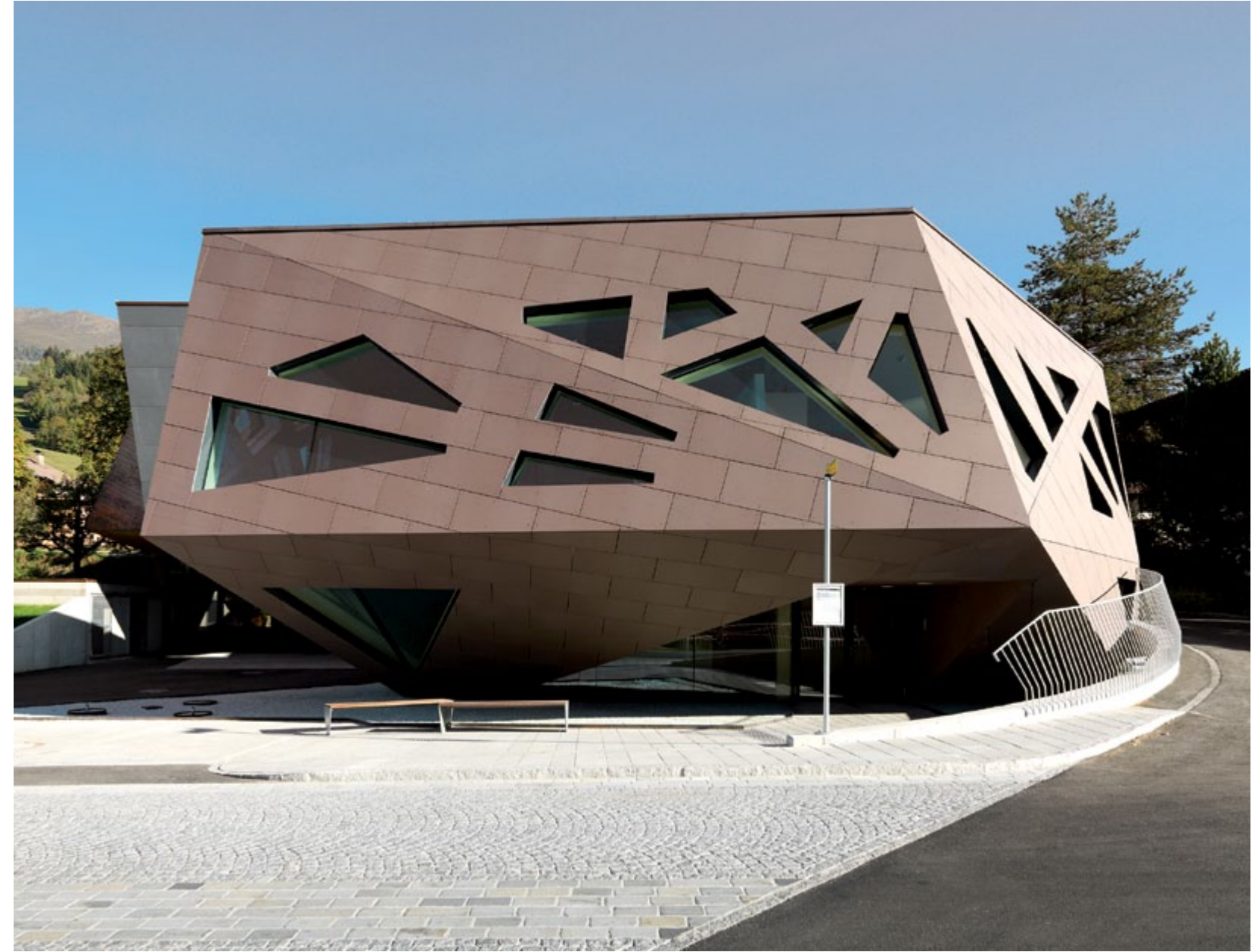
Community Center Abfaltersbach, AT | Machné Architects Innsbruck, AT | 1,000 m 2 fibreC facade | ivory, silvergrey & mocca brown | FE | screwed
