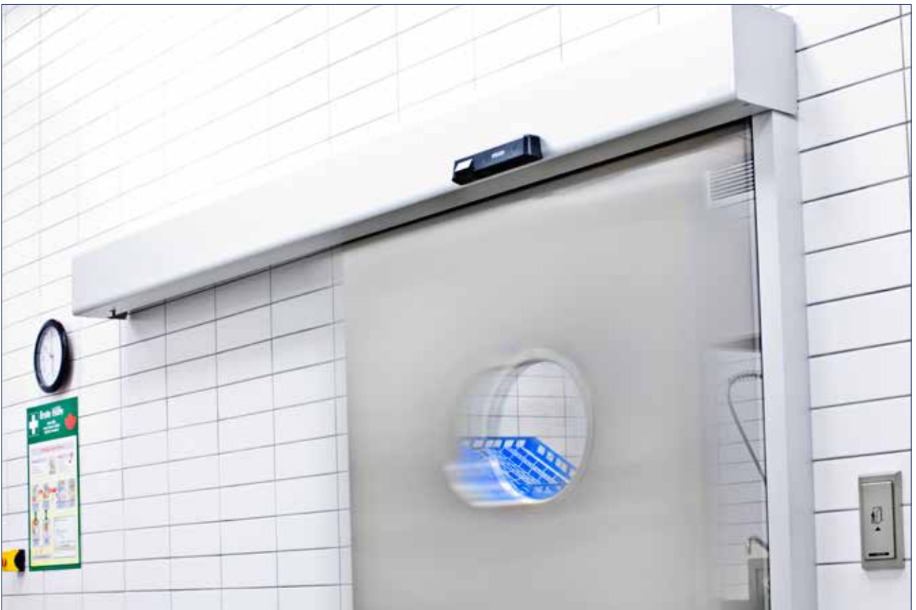
Automazione Powerdrive, VGH Assurances, Hannover, Germany (Photo: Lothar Wels)
