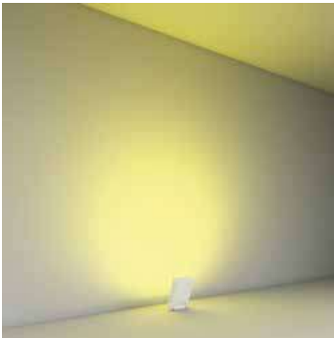
Installation on floors/walls, wall washer.
