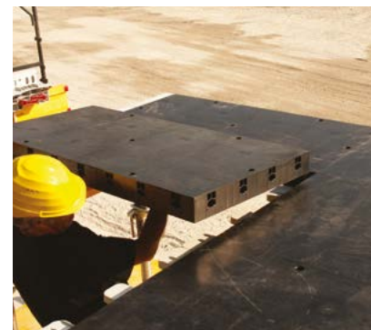
③ POSA PANNELLI GEOPANEL
